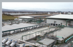
Ringsend Sludge Treatment Plant Extension /23
