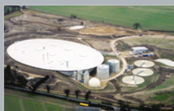
Lowestoft Wastewater Treatment Plant /20
