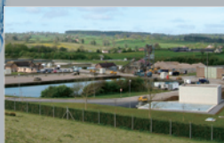
Barrow Water Treatment Plant /19
