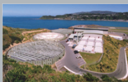
Moa Point Wastewater Treatment Plant /21
